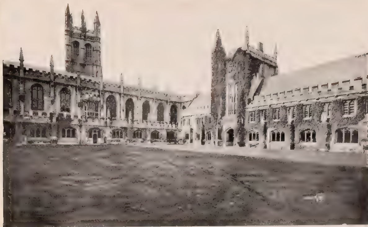
Cloisters and Tower, Magdalen College, Oxford
